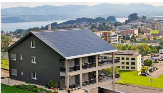
Apartment house with photovoltaic system
